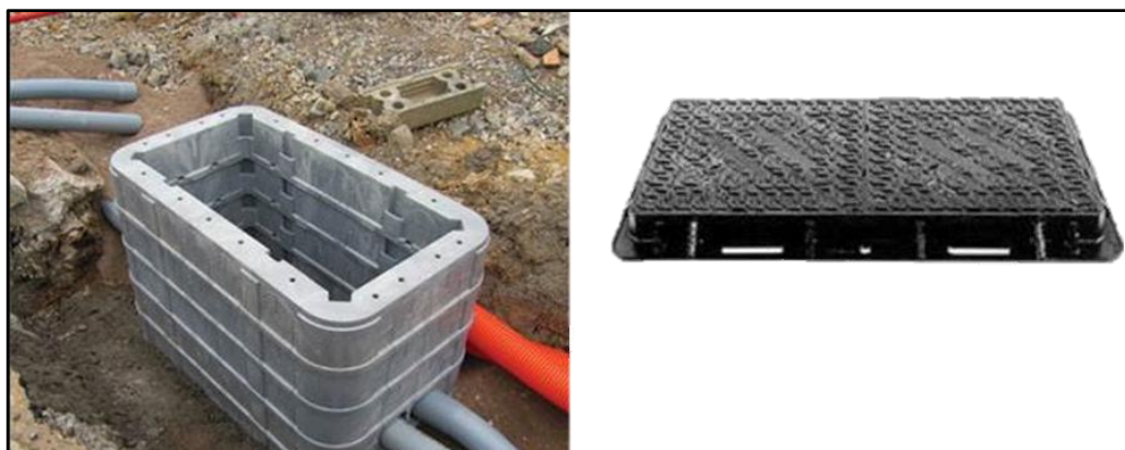
Plate 12 Fibre Chambers (construction and external appearance)
