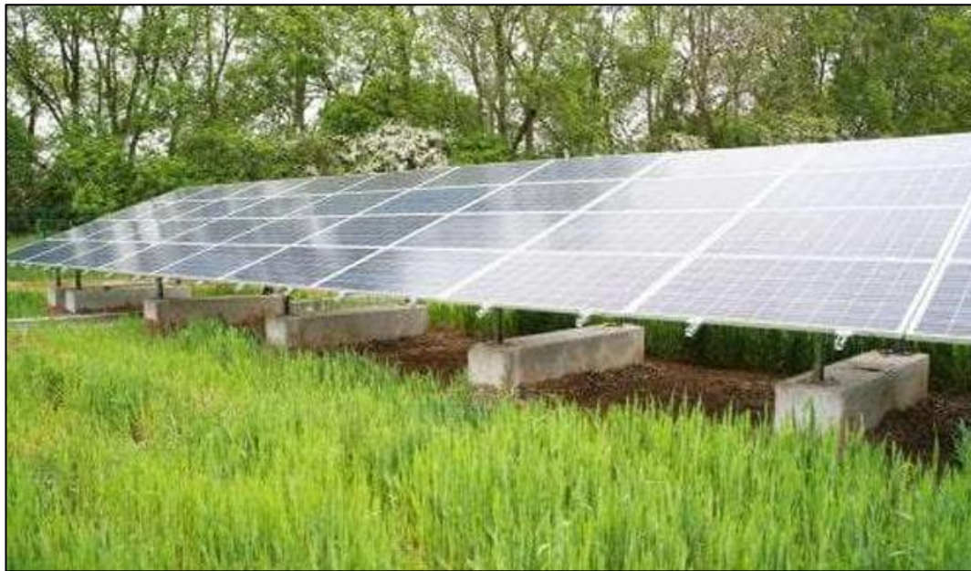
Plate 4 Fixed Panels on Concrete Feet
