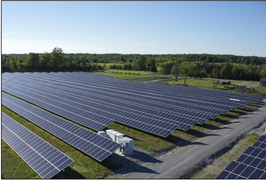
Plate 5 Typical Fixed South Facing Arrays (with Conversion Unit/Inverter) 33kV Sub-distribution Switch Rooms
