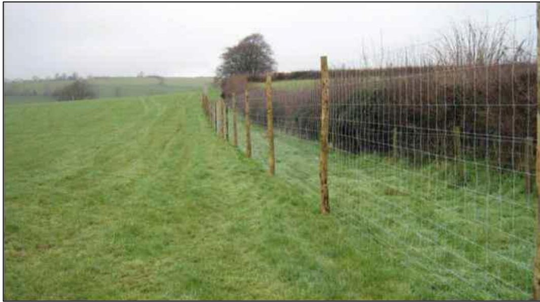
Plate 13 Typical Deer Fencing
